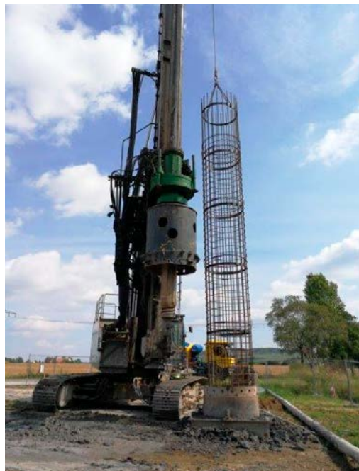
Illustrative photos of reinforcement cage/drilling situation
