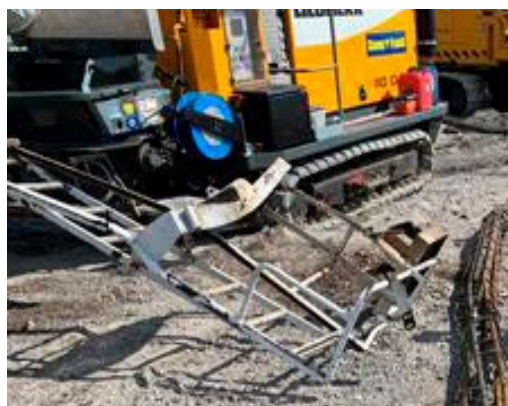
Damaged excavator and reinforcement cage
