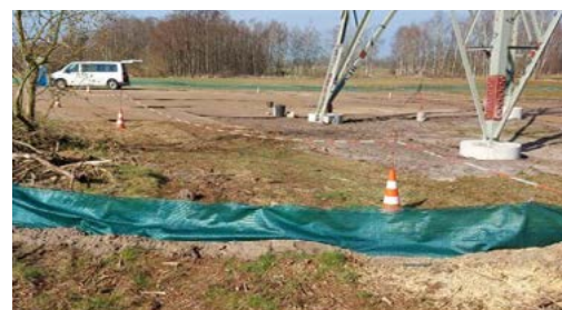
Figure 5: Example of how to demarcate a drop zone
