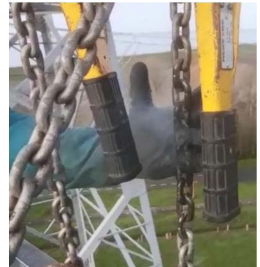
Heating (smoke/vapour formation) of chain hoist due to not properly functioning earthing for work. The chain hoist is suspended here with a steel stop. If the chain hoist had been suspended with a plastic (insulated) stop, no current could have passed through so there could also have been no heating.
