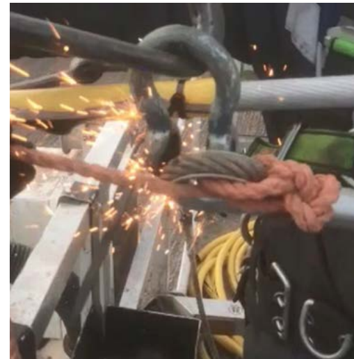
Sparks due to not properly functioning earthing for work. This involves two separate live parts earthed on 1 side (bow shackle and steel cable) so a voltage difference originates in both parts (they are never equally long). Because both parts are held against each other, the voltage difference wants to equalise, with the formation of sparks as a consequence.
