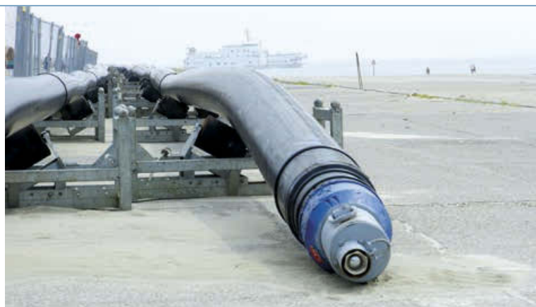
Horizontal boreholes: The actual cables are pulled through the plastic pipes later.
