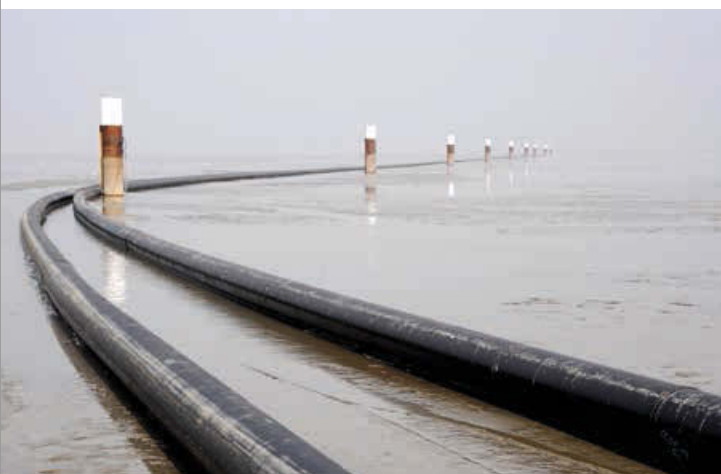
To protect dykes, dunes and the Wadden Sea, TenneT carries out horizontal directional drillings. First, protective conduits are pulled into the borehole. In a second step, the high voltage cables are being pulled into the conduit.
