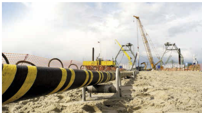
During the cable pull-in the cables are positioned on cable roller tracks.
