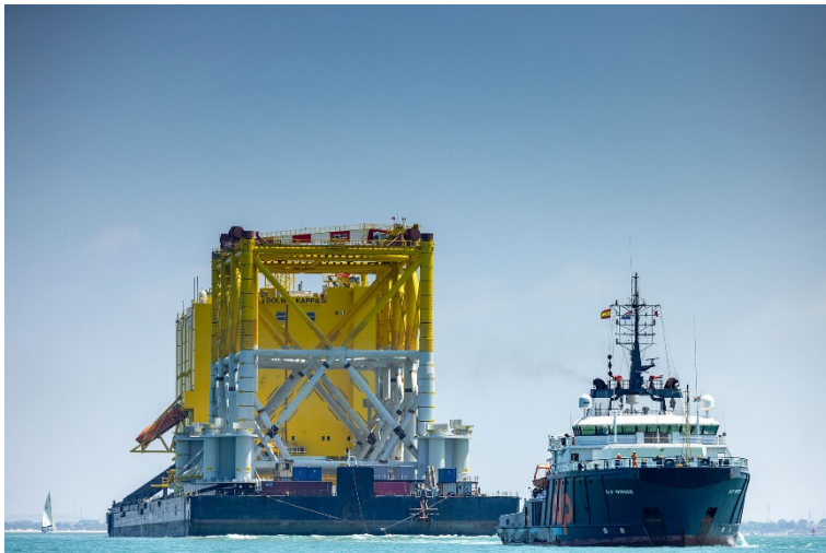
(Picture 20220805_TenneT_DolWin-kappa_Sailout_Low-Res_01-04: Sail-out of offshore converter station DolWin kappa; Photo Credit: © TenneT)
